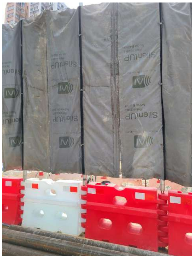
Figure A1 Noise barrier mat erected along site boundary
